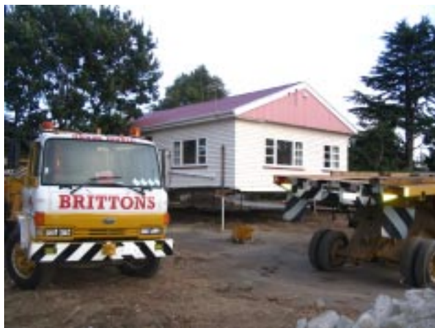
No. 7 Blair street on the move, with final placement taking care to protect surrounding trees.
